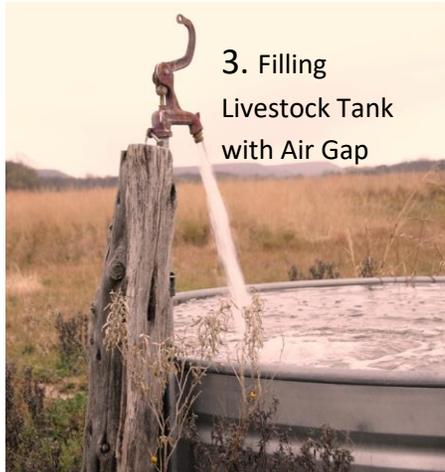
3. Filling Livestock Tank with Air Gap
